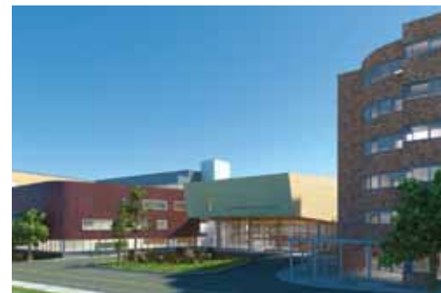
Shore Memorial's Surgical Pavilion includes state-of-the-art operating suites and new recovery and pre-admission areas.
